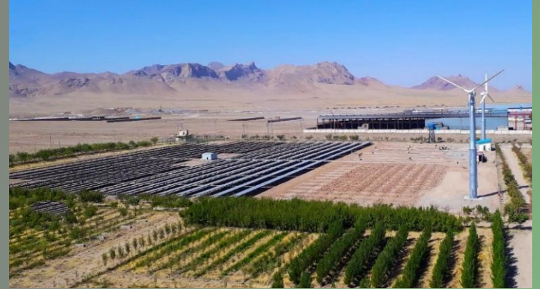
Afghanistan UNOPS 2 MWp
