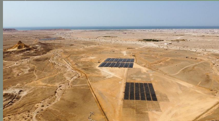
Somalia Bosaso Puntland 3.5 MWp
