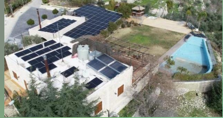
Ghalboun Guesthouse 33 kWp
