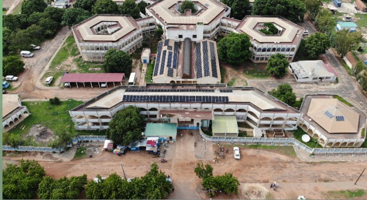
SESCO Gambia 2.2 MWp + 5.4 MWh
