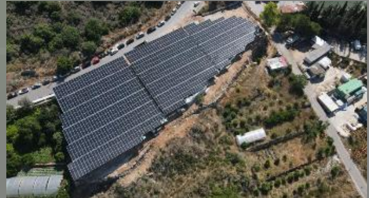
Bellevue Medical Center 750 kWp
