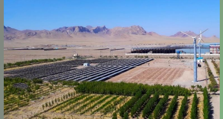
Afghanistan UNOPS 2 MWp
