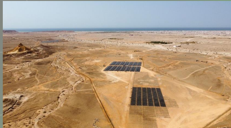
Somalia Bosaso Puntland 3.5 MWp
